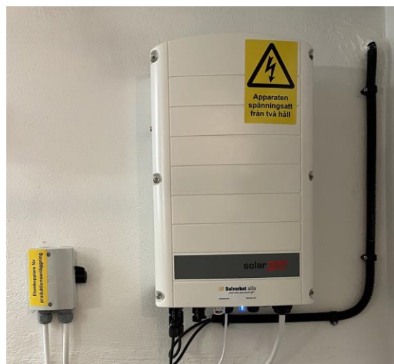
Exempel: Solverket SolarEdge installation brytare
